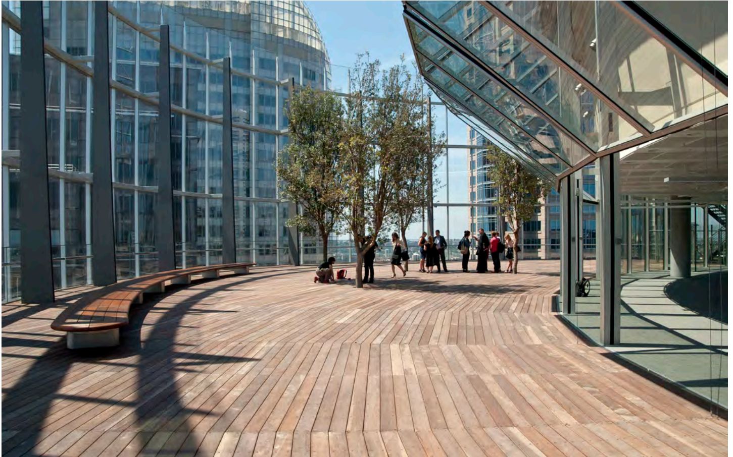
Number 1 Bligh Street's innovative sustainability features include blackwater recycling, trigeneration, solar power and highly efficient double-skin façade
