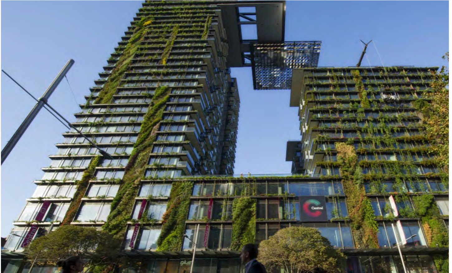
Central Park's stunning green walls are irrigated by water recycled on-site by a private water utility
